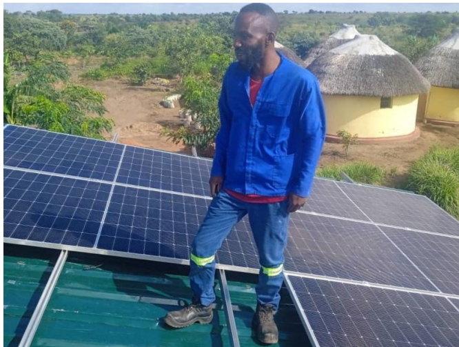
Installing the huge 850W solar panels on the training kitchen roof. The whole of the GAPP site now has solar-generated electricity.
