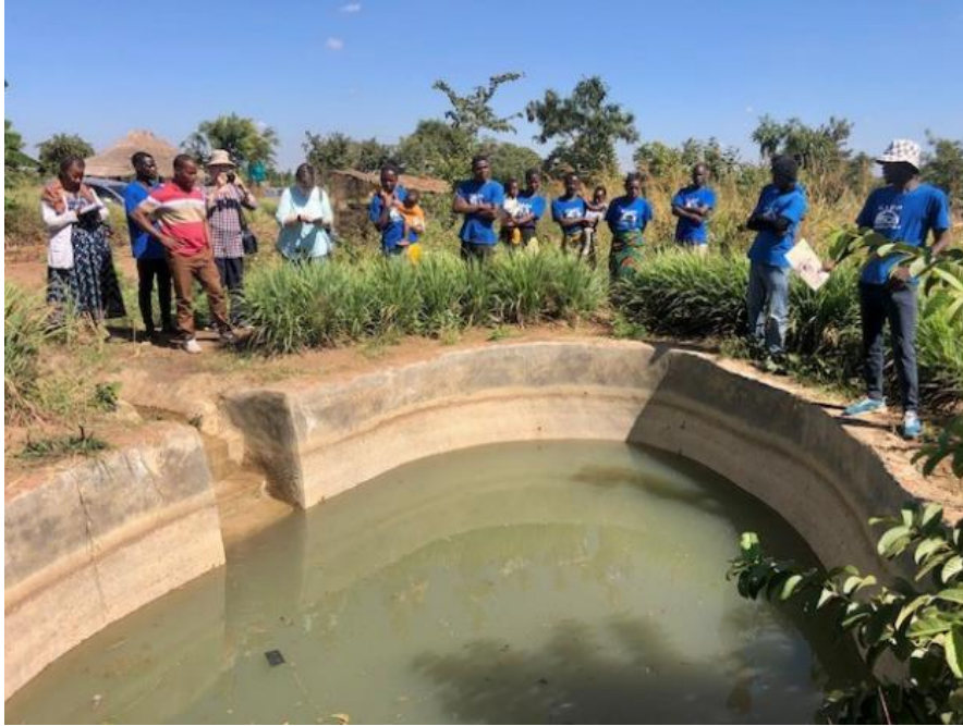
Water Storage Pond - capacity 50,000 litres
